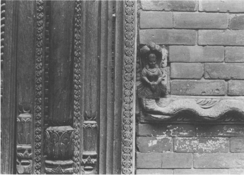
Fig. 4. At close quarters, much of the charm of the older buildings lies in the detailed ornamental carving of their wooden elements. Here a wooden wallband, one of several that encircle the courtyard of Basantpur Chok at various levels, ends in the figure of a Naga, or holy serpent, where it abuts against the elaborate doorframe of the main entrance to the chok.
